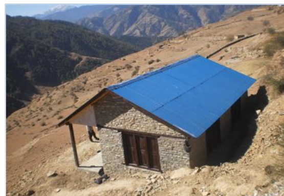
Figure 1 Constructed building of the MBC in Sunnigaun VDC.
